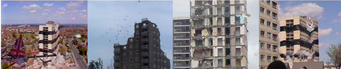
Liverpool demolitions filmed and discussed by tenantspin, 2001-5
